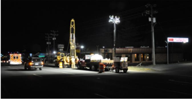
*Drilling and core sampling is being done to determine subsurface conditions before relocation of utilities begins at Rio Road and the Route 29 widening projects.*
